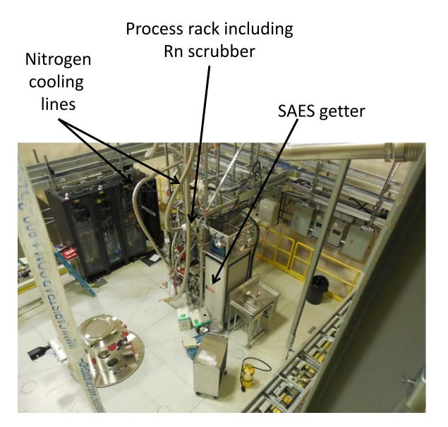
Design of process systems based on minimizing sources of radon:
