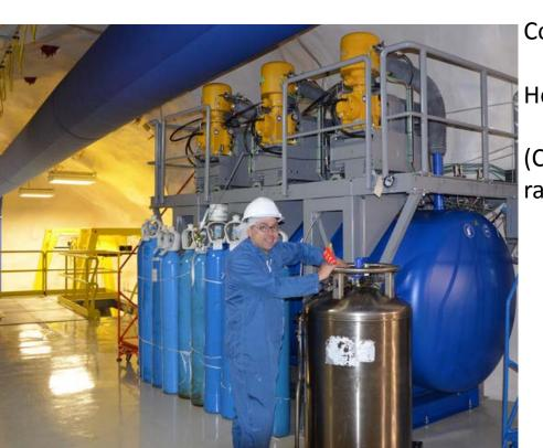
Cooling system: 3kW. Heat load on argon: ≤1kW. (Cooling also required for radon trap.)
